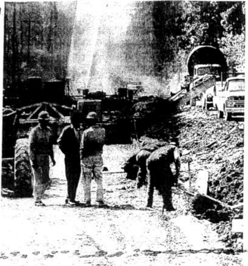
NEARING COMPLETION: The widening of LaGrange Road from two to four lanes between Lyndon Lane and Shelbyville Road is scheduled to be completed by November 15. Curbs and gutters are included in the project which is one mile in length and is costing in the neighborhood of $600,000. The road eventually will be made four lanes wide from Lyndon to Whipps Mill Road.
